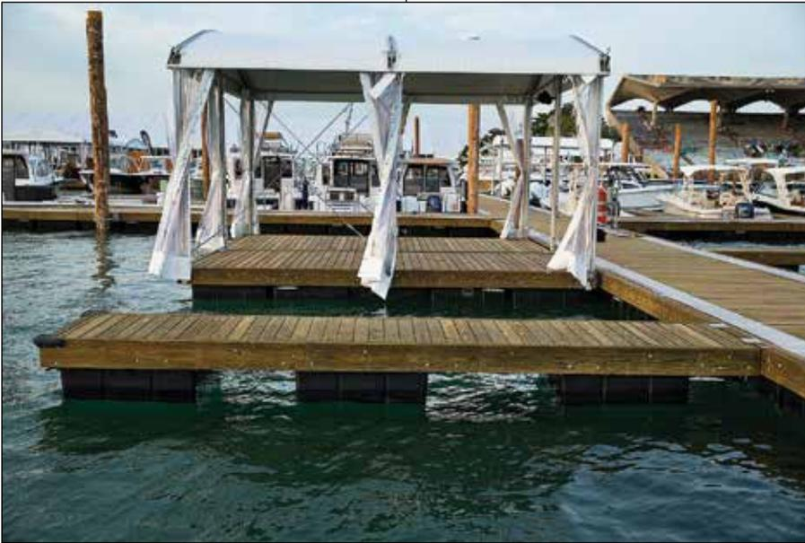
*Bellingham Marine designed and built the docks, including a number of innovative features – recessed cleats, flip-lid utility blocks, hidden lifting eyes, universal connection brackets and more.*
