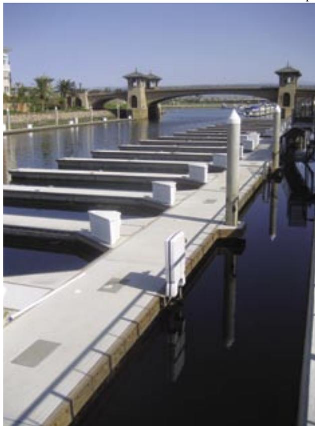
"The individual modules are shorter on the inside and longer on the outside of the curvature," said BMI general manager, Jim Puder. "The dock gets its round, arched appearance from the use of curved concrete forms. We created the tooling and made it expressly for this project."
