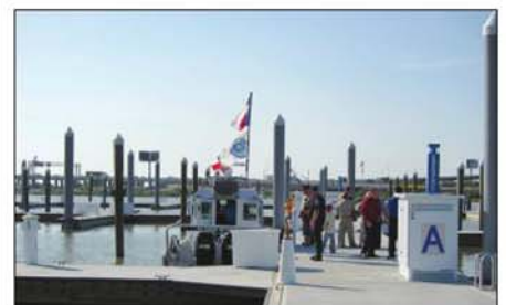
The new configuration at Bayland Marina is more wave resistant and provides easier access in and out of the marina.
