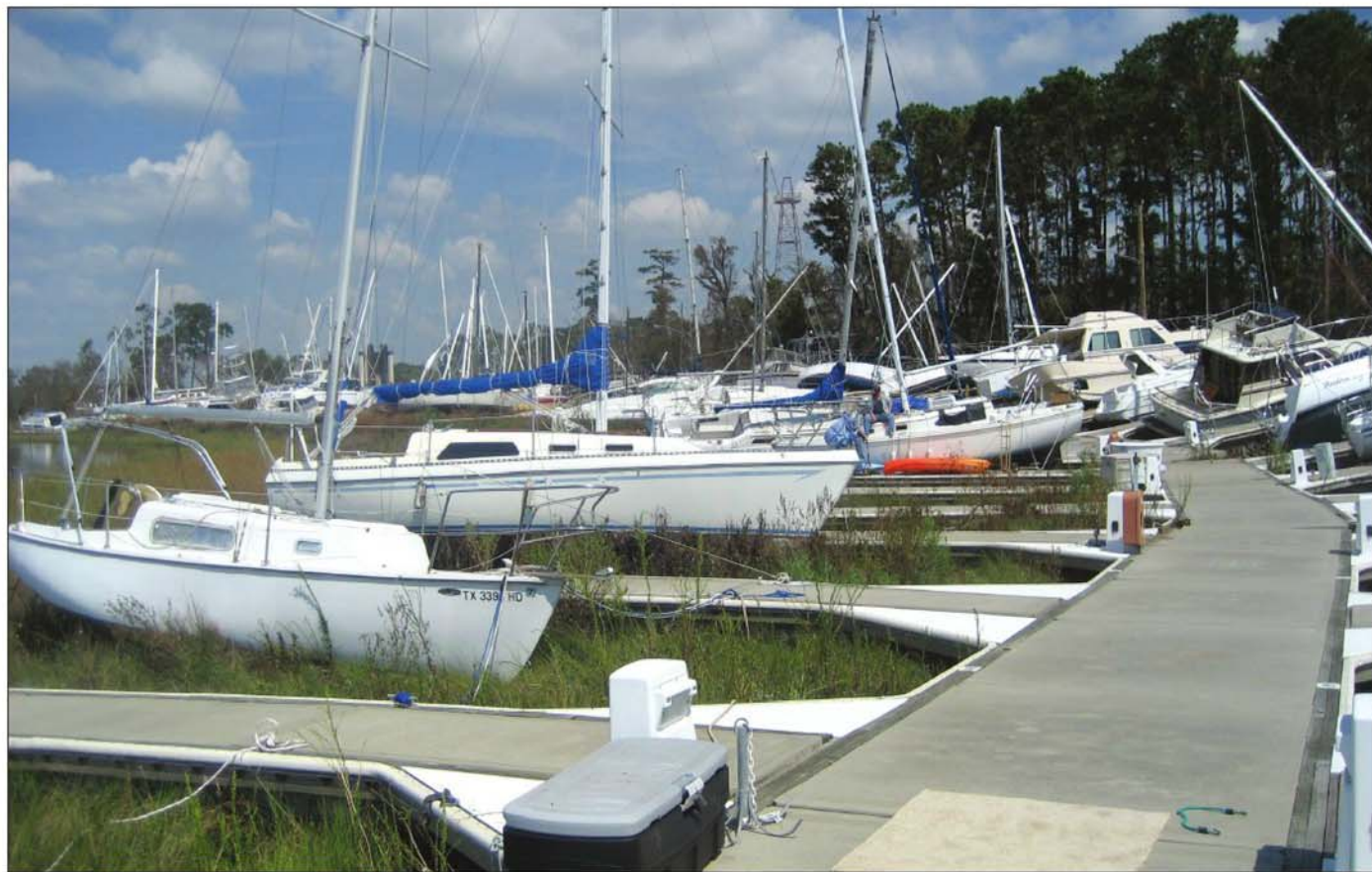
When Hurricane Ike hit Bayland Marina in Baytown, Texas, the marina was lifted above the pilings and floated inland until it was stopped by the tree line. The cleanup began six weeks after the storm, and six months before the last boat was craned into the water.
