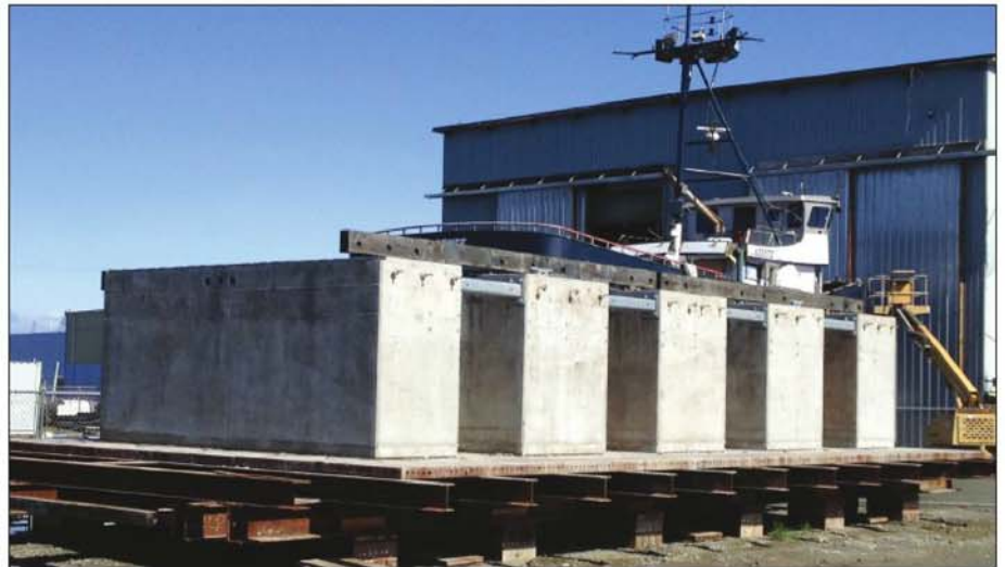
This module for the outer dock at Crescent City shows pre-installed pockets in the dock for the piling.
