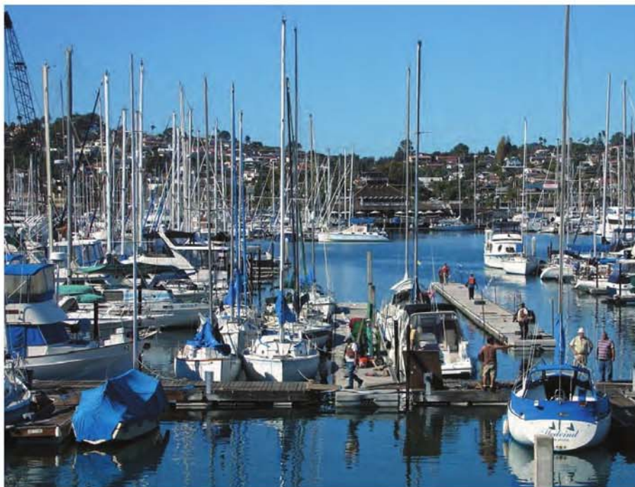
As part of the renovation, workers get ready to move the concrete floating docks into place at the marina. Credit: Bellingham Marine
