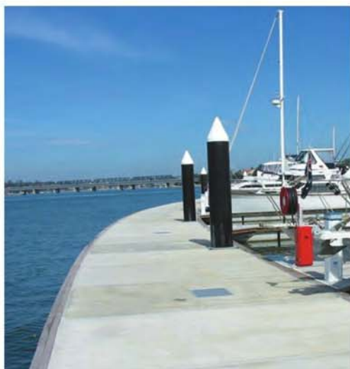
This wave attenuator's curved shape aids in wave energy absorption and diminishes the reflected wave.
