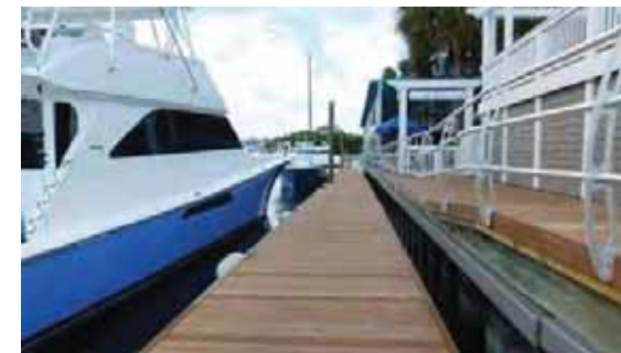
lpe hardwood decking, timber frame.
