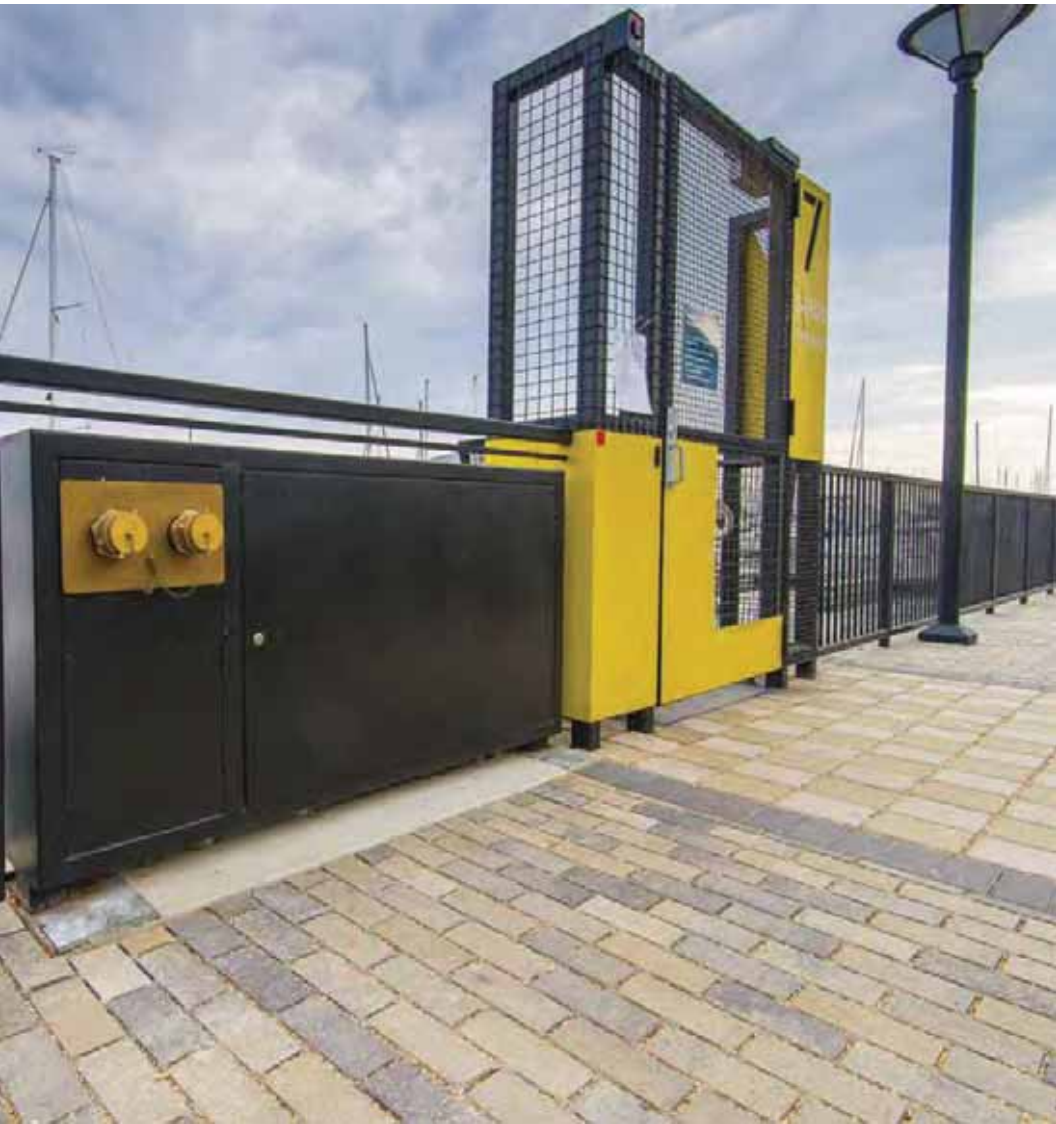
Metal railing and security gate, Harbor at Marina Bay
