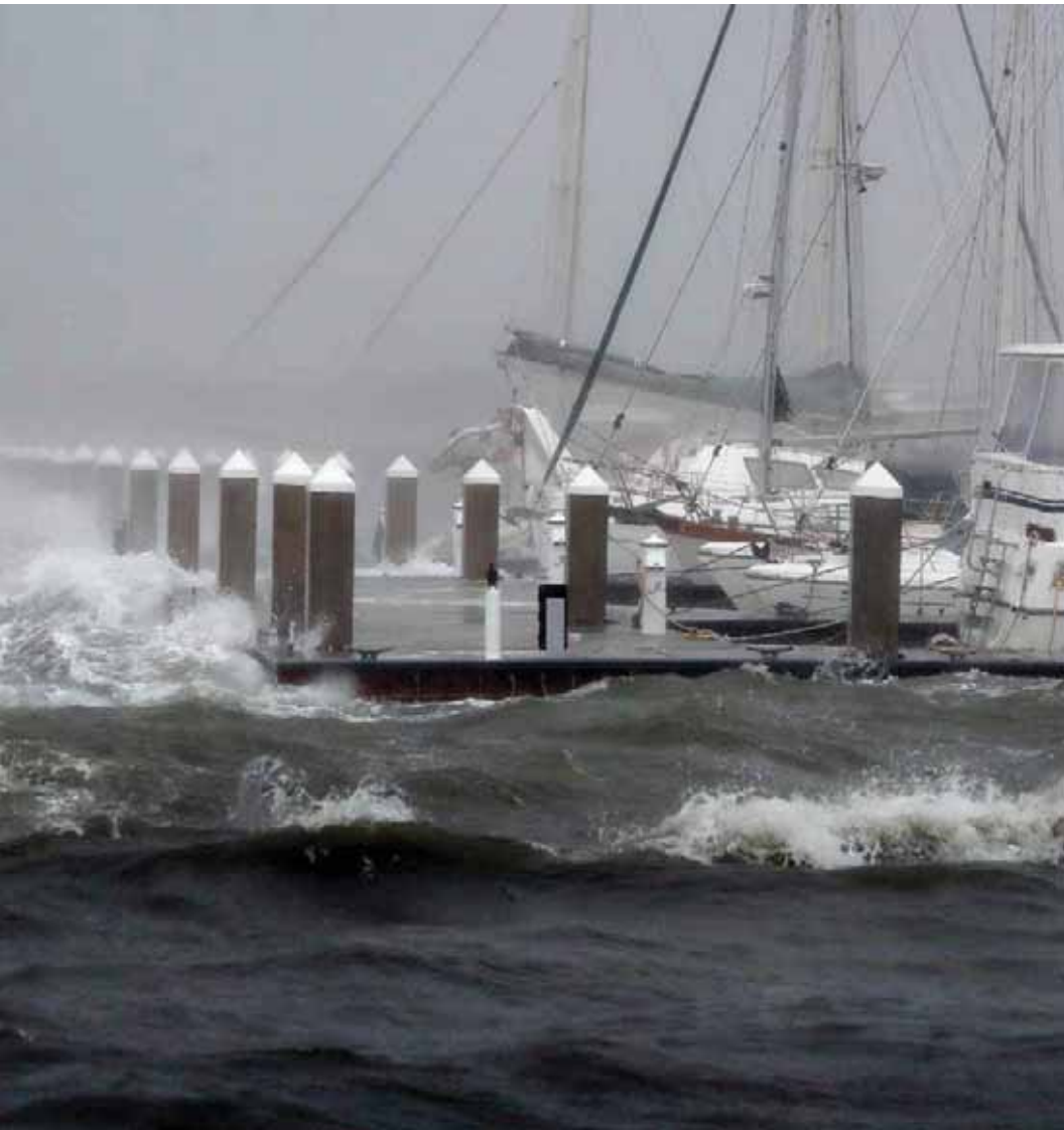
St. Augustine's wave attenuator during Hurricane Matthew
