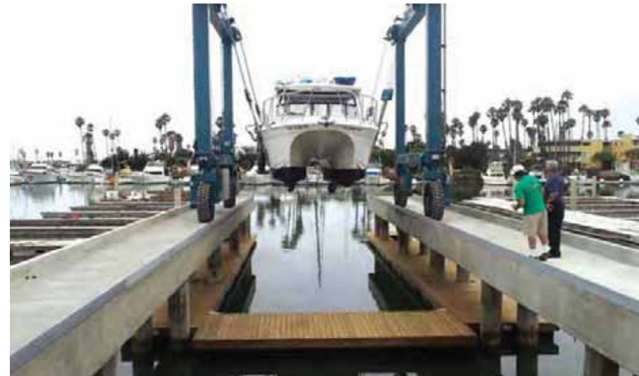
Travel-lift pier with timber service docks, Channel Islands Boatyard
