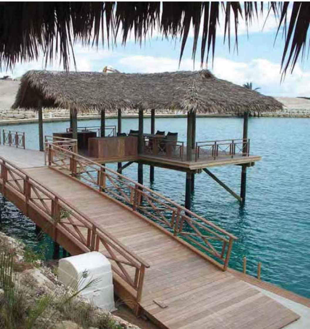
Fixed access pier and cabana, private marina in the Bahamas.
