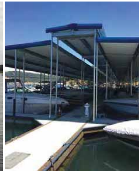
Covered Unifloat concrete docks
