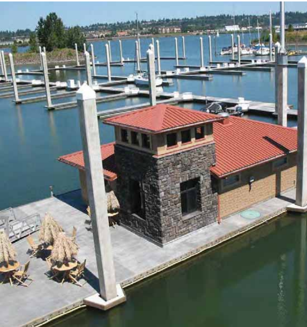
Marina office and public outdoor space, Salpare Bay Marina
